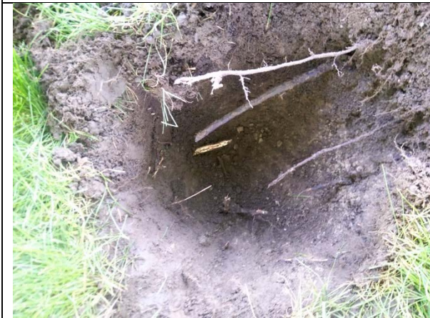
IMAGE 3 VIEW OF TEST PIT IN PROGRESS
