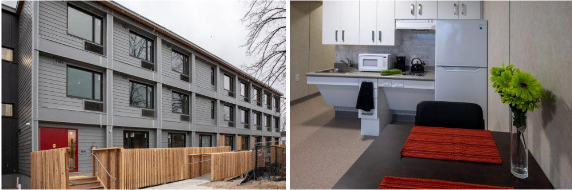
Figure 22: Exterior and Interior Finishes of a Modular Building at 321 Dovercourt Road in Toronto
