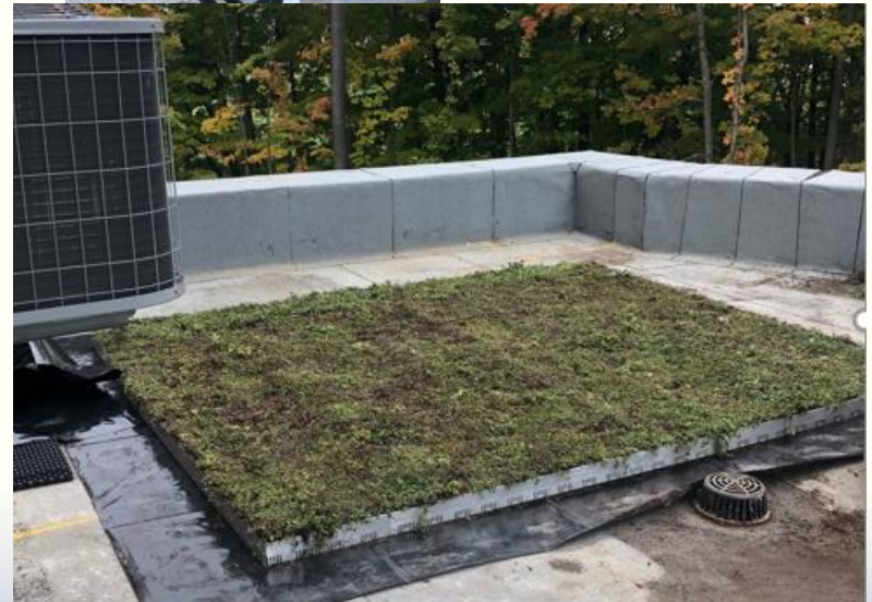
Photo: Victoria Harbour green roof installation
