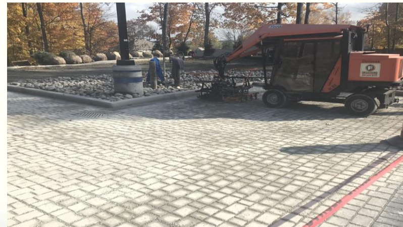
Photo: Victoria Harbour permeable pavers installation
