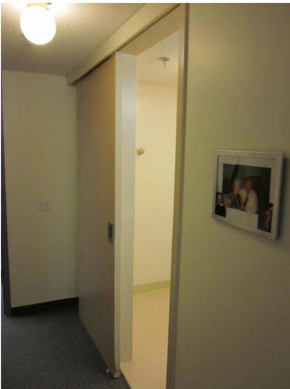
Image 6: Interior Conditions – Dated Suite
