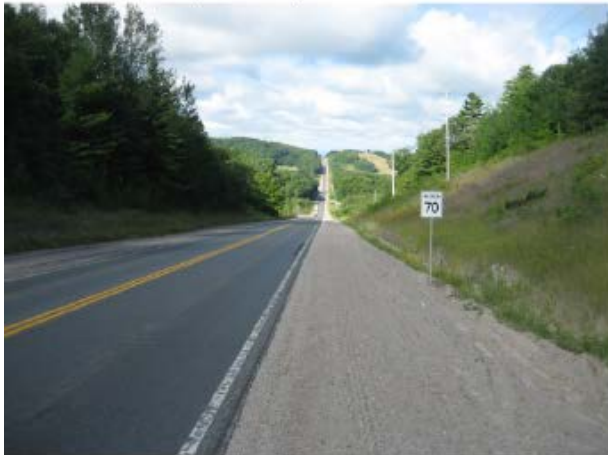
Plate 15. Disturbed Road Corridor, 400m West of Line 4 North (view west)
