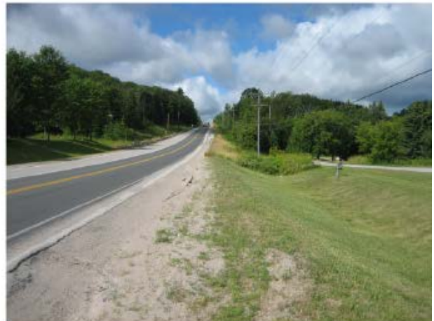
Plate 10. Disturbed North Side of Corridor, Immediately West of Entrance to Horseshoe Valley Resort (view west)
