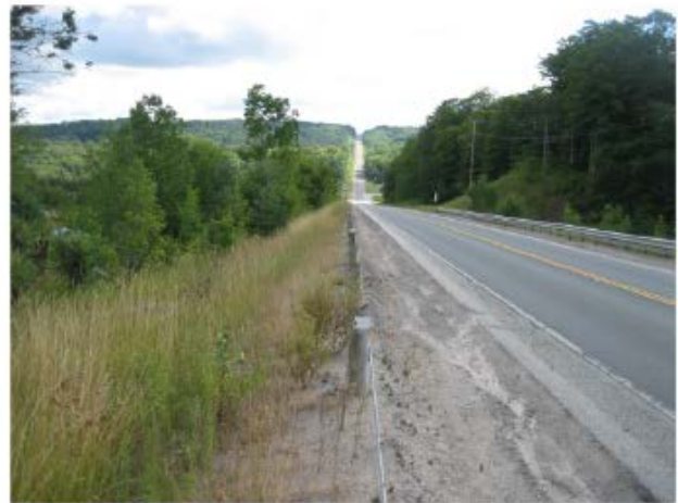
Plate 6. Disturbed North Side of Corridor, 500m West of Entrance to Horseshoe Valley Resort (view east)
