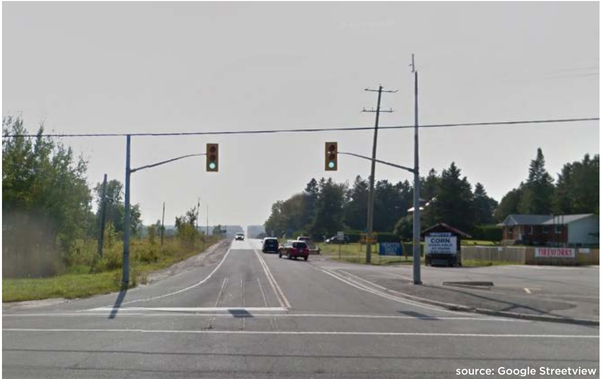
Looking west along County Road 22 from Highway 12
