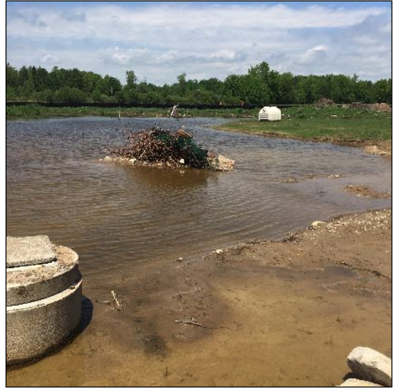
Image 6: Area of extensive disturbance via grading.
