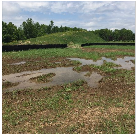
Image 4: Area of disturbance and grading in the foreground; spoil heap in foreground.
