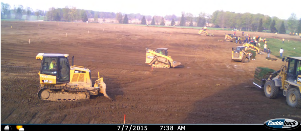
Image 12: Area of disturbance from topsoil grading, facing southwest, photo provided by client.
