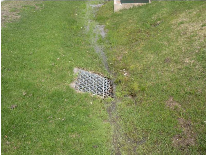
PHOTOGRAPH 5. Grate in south ditch of Millwood Road conveying flow into pipe buried within adjacent park (May 8, 2017)).
