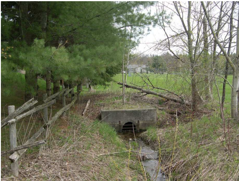
PHOTOGRAPH 6. Outlet of mapped drainage feature at north end of park (May 8, 2017).
