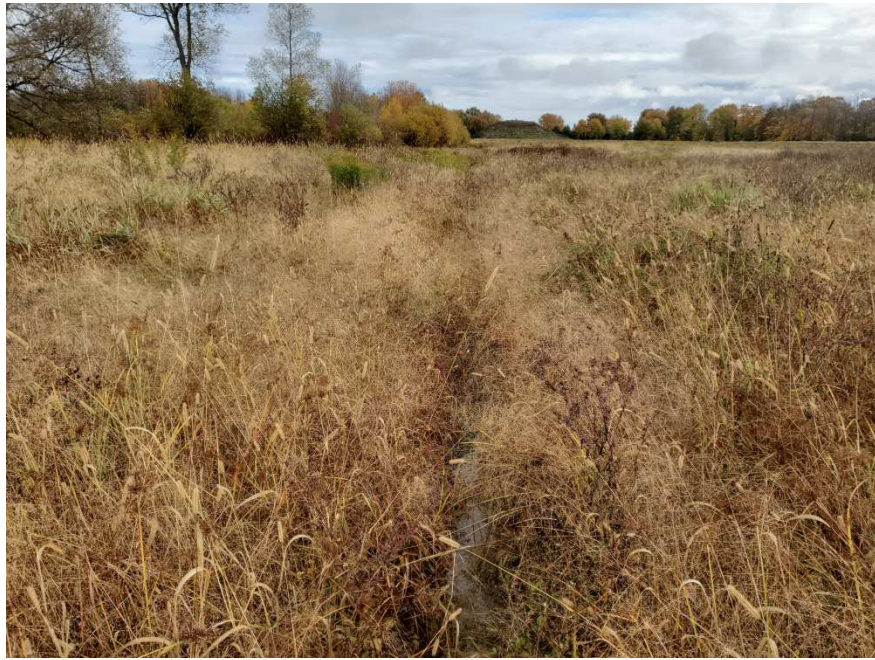
Photograph 1 – Drainage ditch on property, facing northeast (October 16, 2020).
