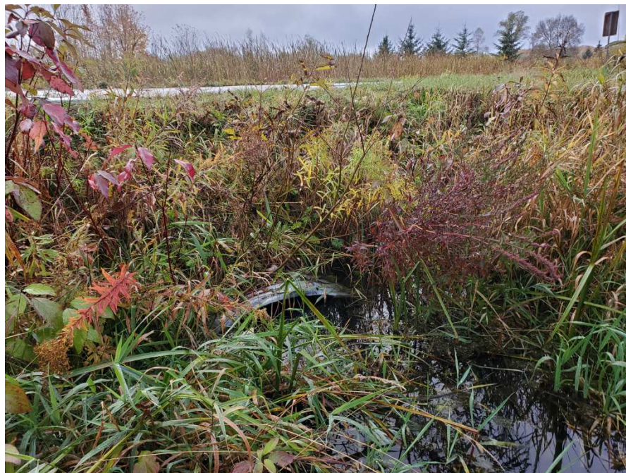
Photograph 8 – Amigo Drive culvert outlet (October 16, 2020).
