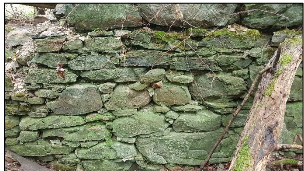
Figure 24: Detail view of stone foundations (ASI 2018).
