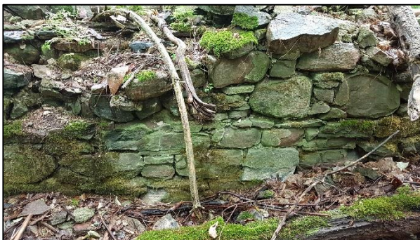
Figure 23: Detail view of stone foundations (ASI 2018).
