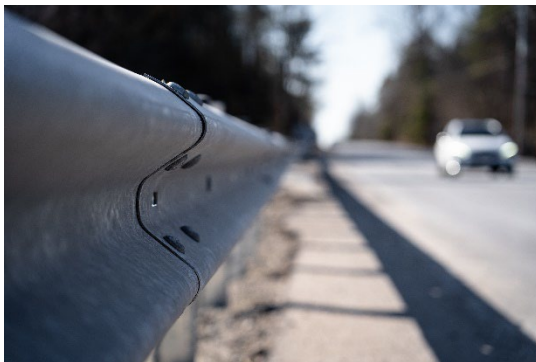
County Road 56 Guide Rail
