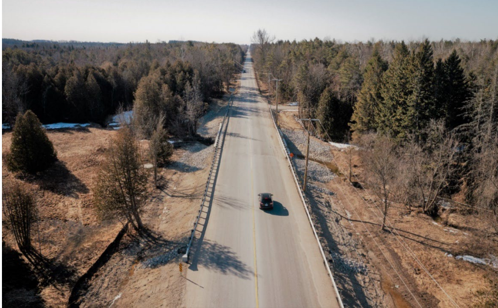
County Road 56 – Concession 6/7 Lot 24 Culvert
