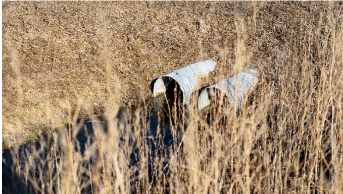
County Road 21 Stormwater Outlet
