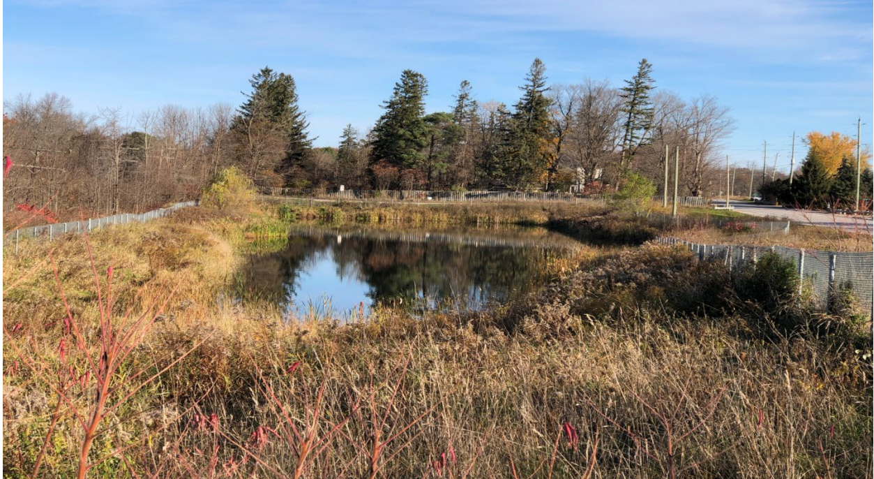
Stormwater Pond - County Road 44 CN Drainage Across from Fowlers Pit
