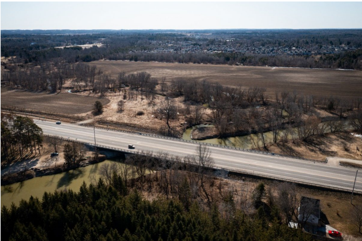
County Road 90/Mill Street - Elliot Bridge over Nottawasaga River
