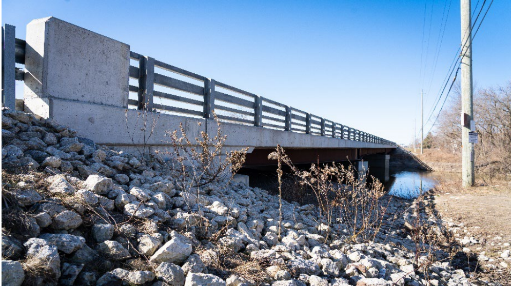
County Road 90/Mill Street - Elliot Bridge over Nottawasaga River
