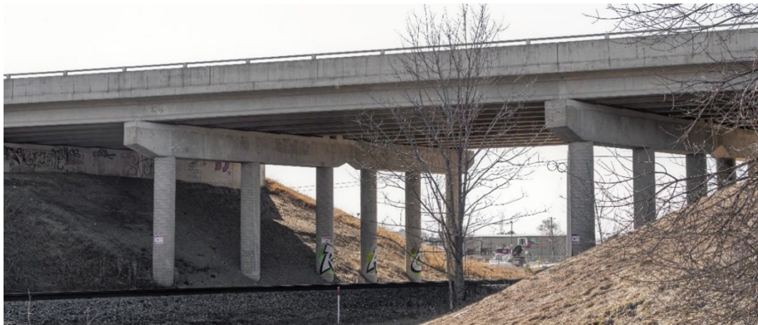
County Road 90 – CPR Overhead Bridge - Slab on Concrete I Girders
