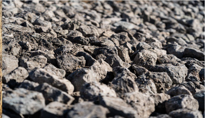
Infiltration Ditch Rocks
