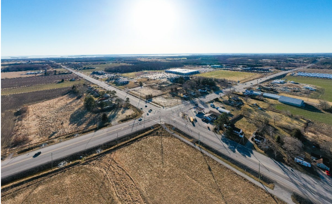
Intersection of County Road 21 & County Road 4 (Innisfil Beach Rd. & old Hwy. 11)
