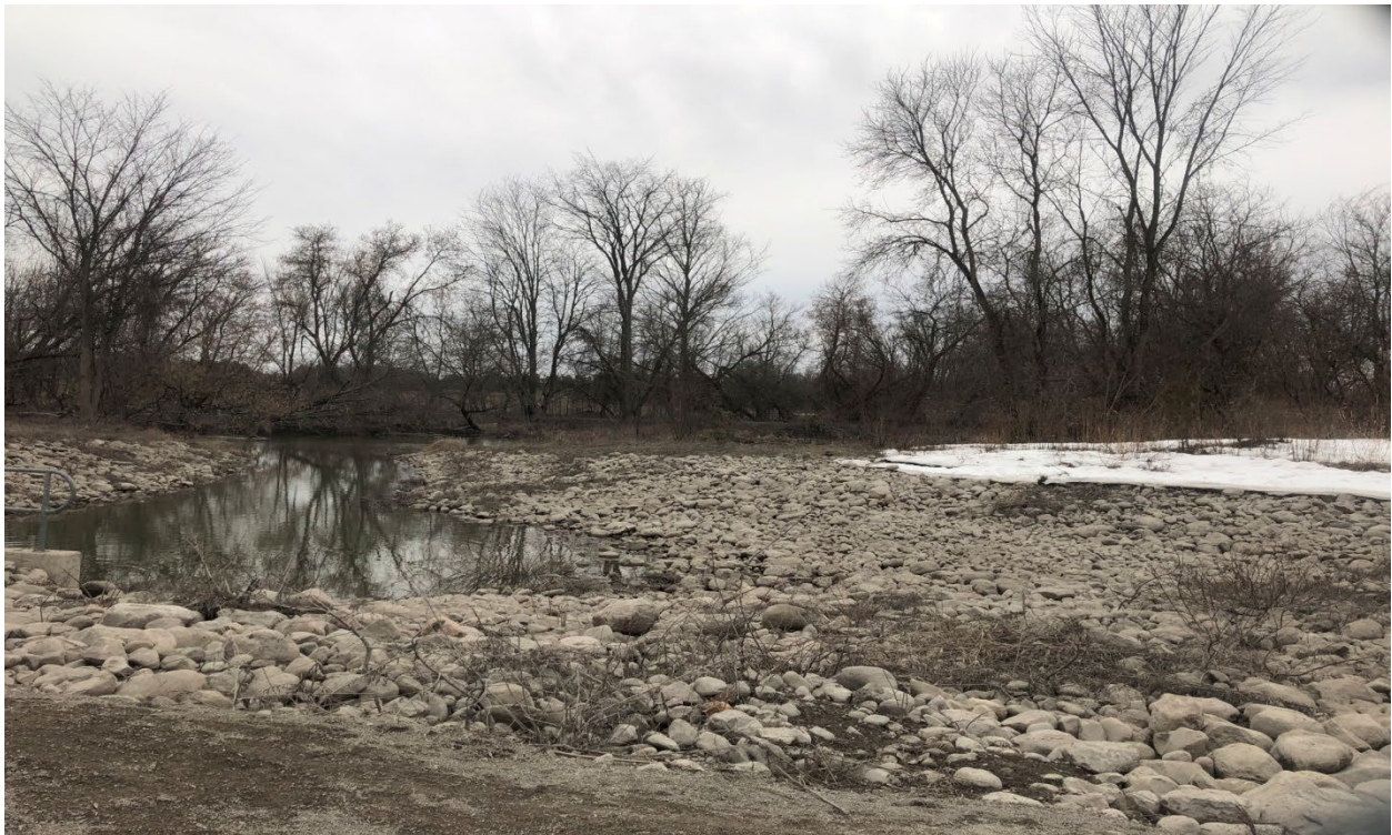
Stormwater Pond Outlet- County Road 90 at McKinnon Road outlet to Pine River
