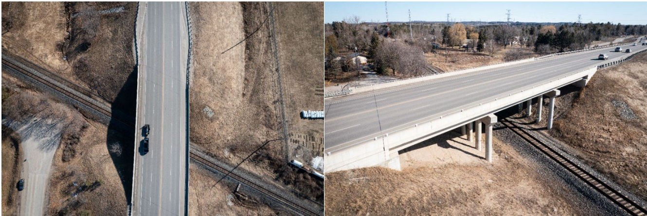
County Road 90 – CPR Overhead Bridge - Slab on Concrete I Girders
