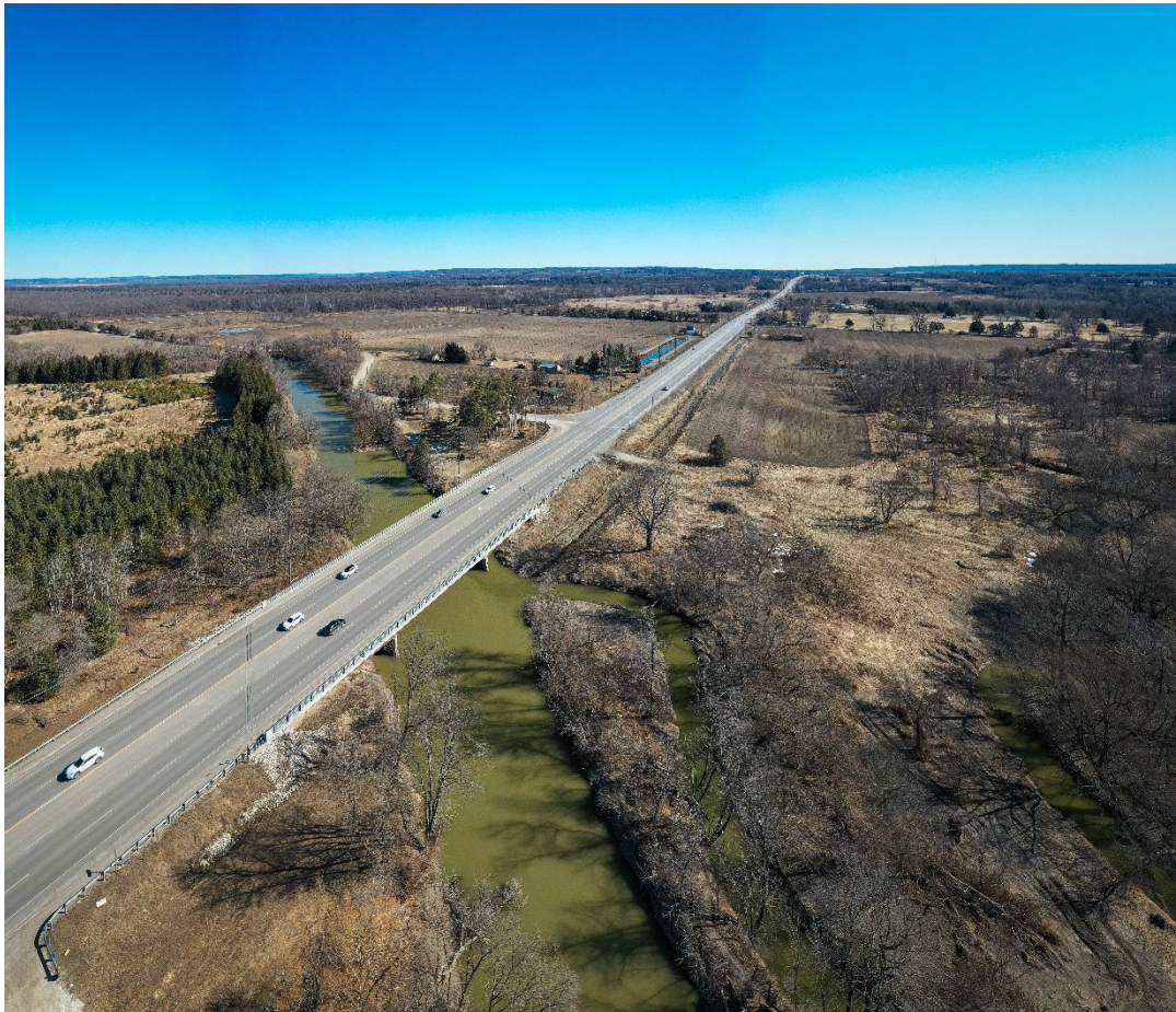
County Road 90/Mill Street - Elliot Bridge over Nottawasaga River
