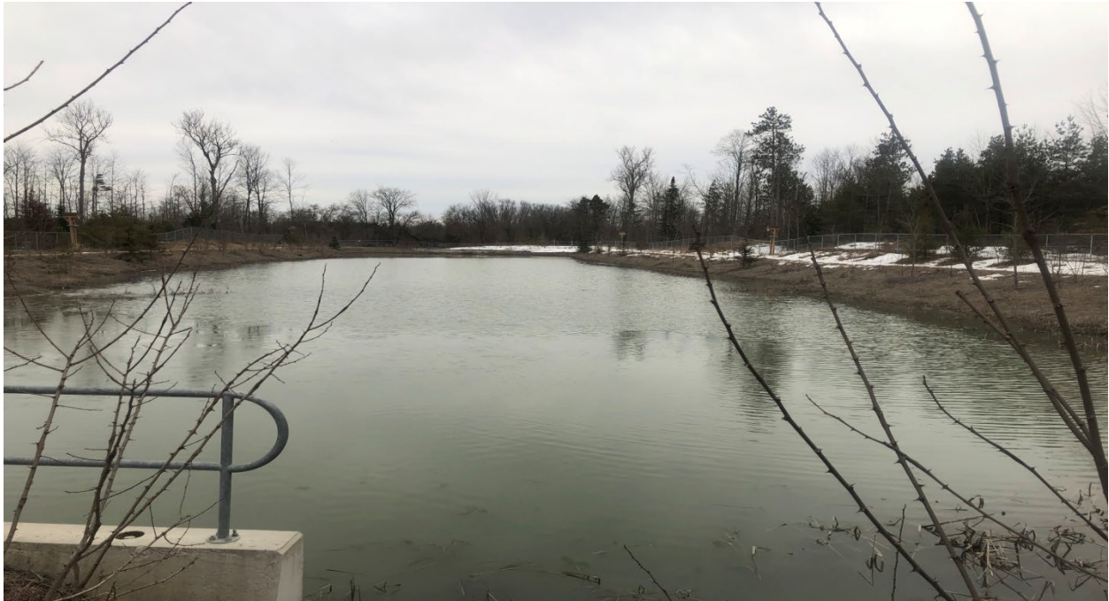
Stormwater Pond - County Road 90 at McKinnon Road
