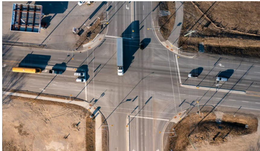
Intersection of County Road 21 & County Road 4 (Innisfil Beach Rd. & old Hwy. 11)
