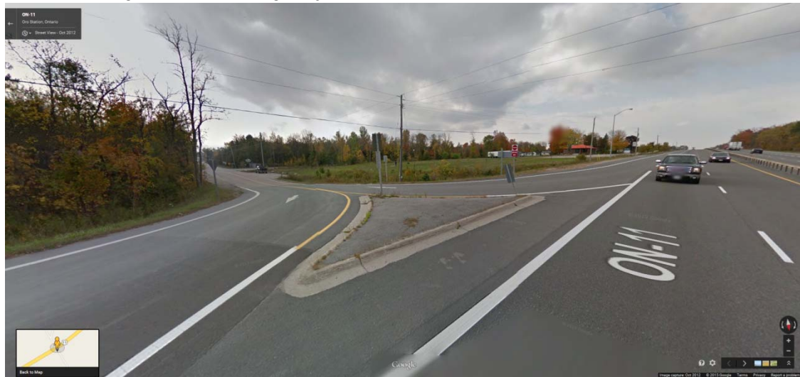
Highway 11 NB looking towards Line 8 right-in/right-out
