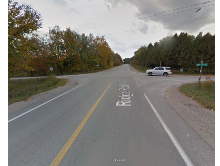
Simcoe Road 20 looking south at Line 9
