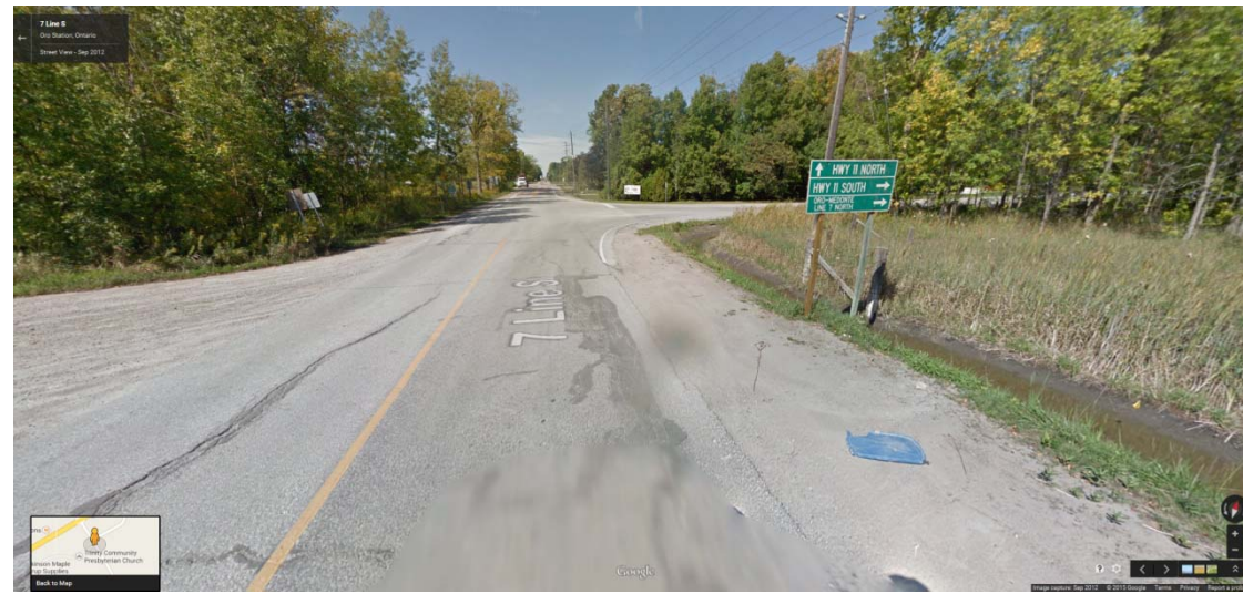
Line 7 looking west towards Highway 11 overpass intersection
