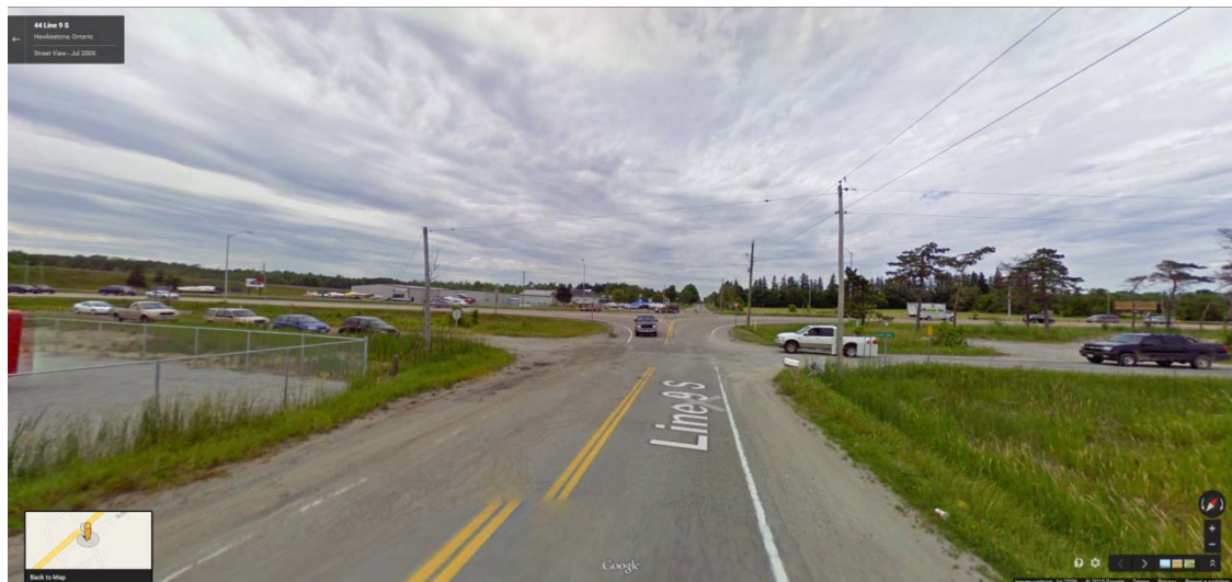
Line 9 looking west towards Highway 11
