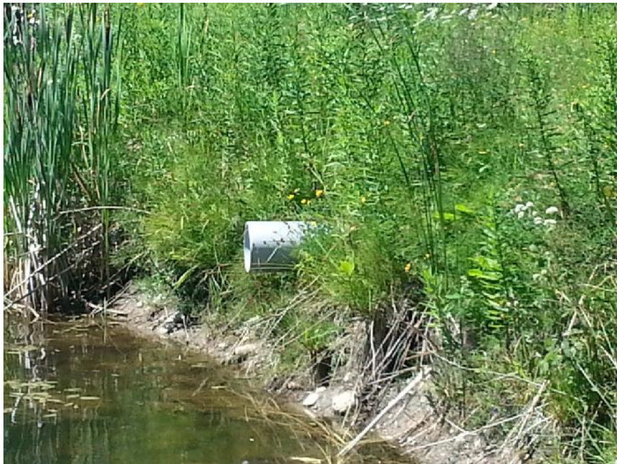
Photo 10. SWM Pond 2, north arm. Photo of culvert inlet from north.
