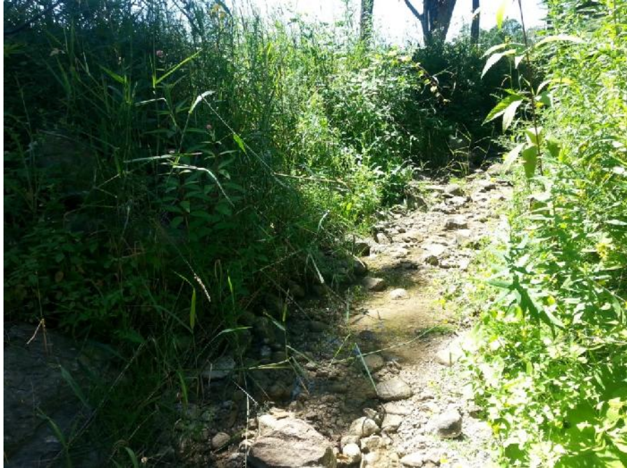
Photo 41. Burl's Creek, photo facing upstream from Culvert 4.
