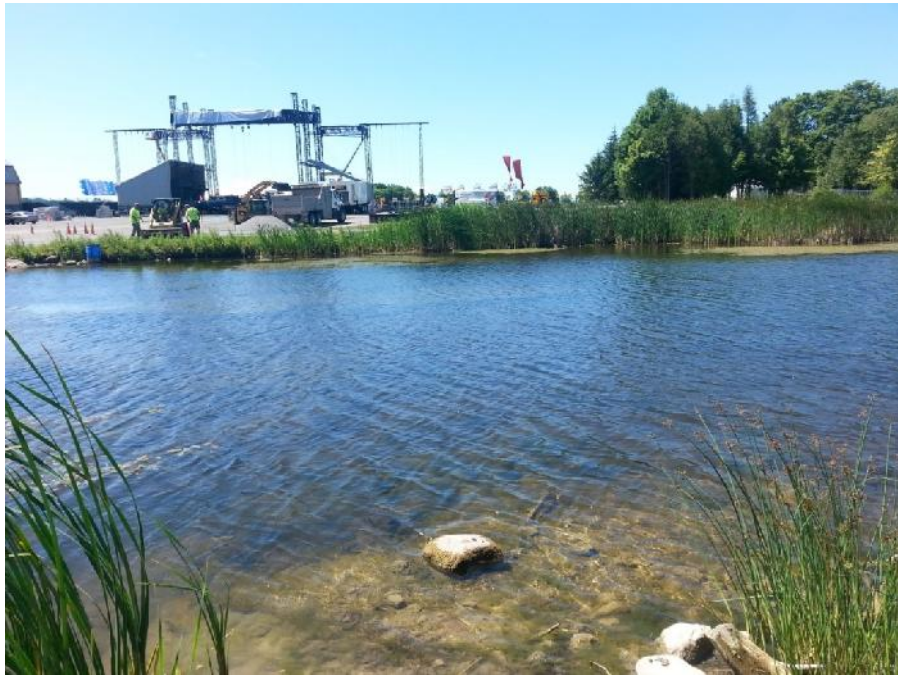
Photo 4. SWM Pond 2. Photo from east facing west.
