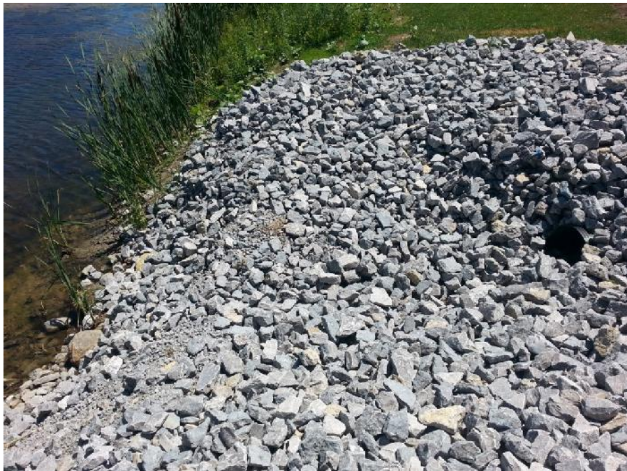
Photo 12. SWM Pond 2. Photo of inlet on west bank.
