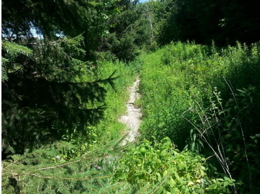
Photo 43. Burl's Creek, photo facing downstream from Culvert 4.
