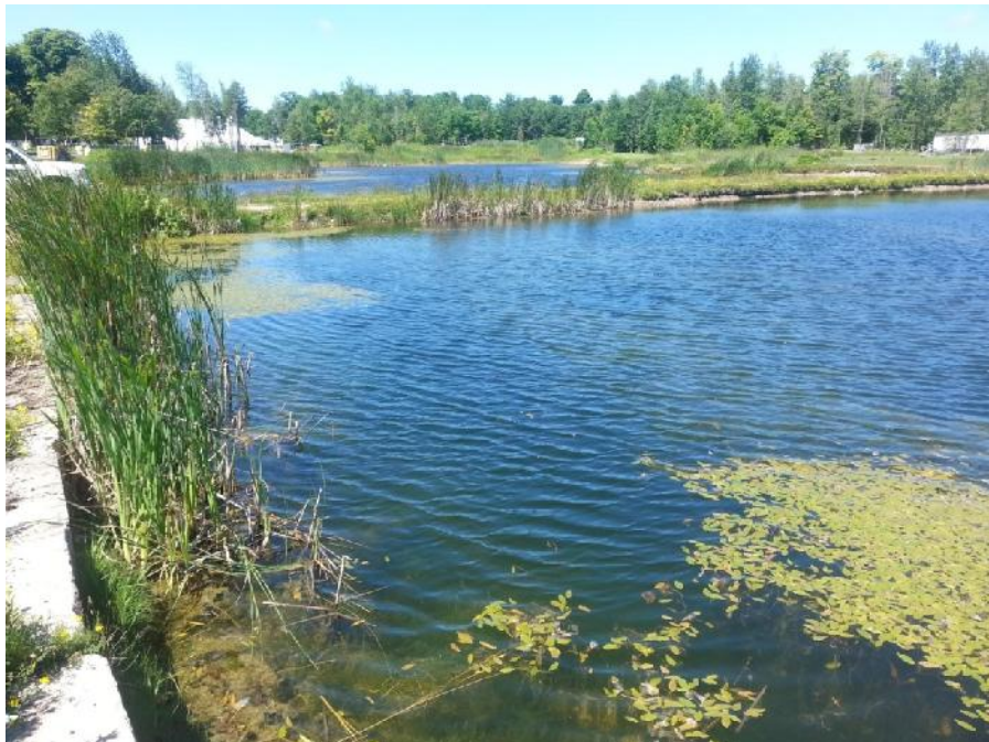
Photo 2. SWM Pond 1. From south facing west, showing south engineered concrete block bank and western gravel causeway with naturalized bank.
