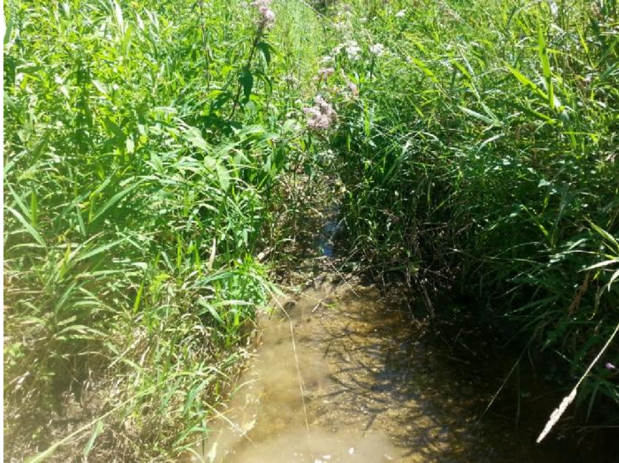
Photo 39. Burl's Creek. Downstream view from Twin Culverts 3a and 3b.
