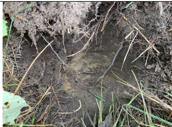
IMAGE 4 SAMPLE TEST PIT IN PROGRESS
