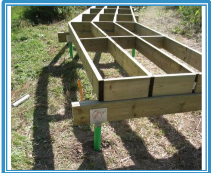
Boardwalk Examples- Hamilton, ON (left) & Boardwalk Foundation on Helical Piles (Halton Hills) (right) Credit: MMM Group
