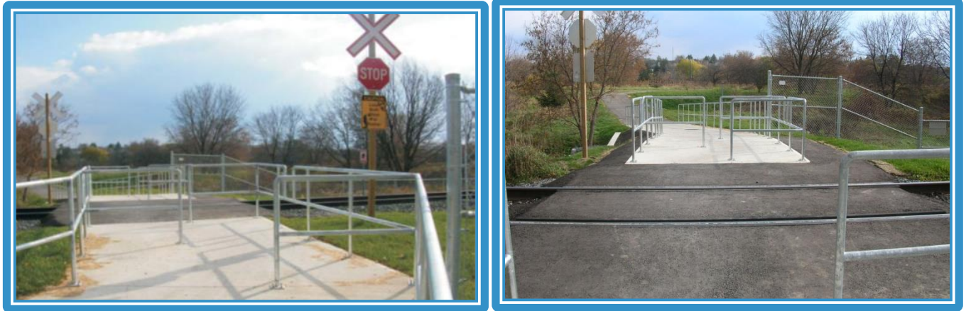
At-Grade Trail Crossing of a Railway - Location: Newmarket, ON Credit (Right / Left): MMM Group, 2012
