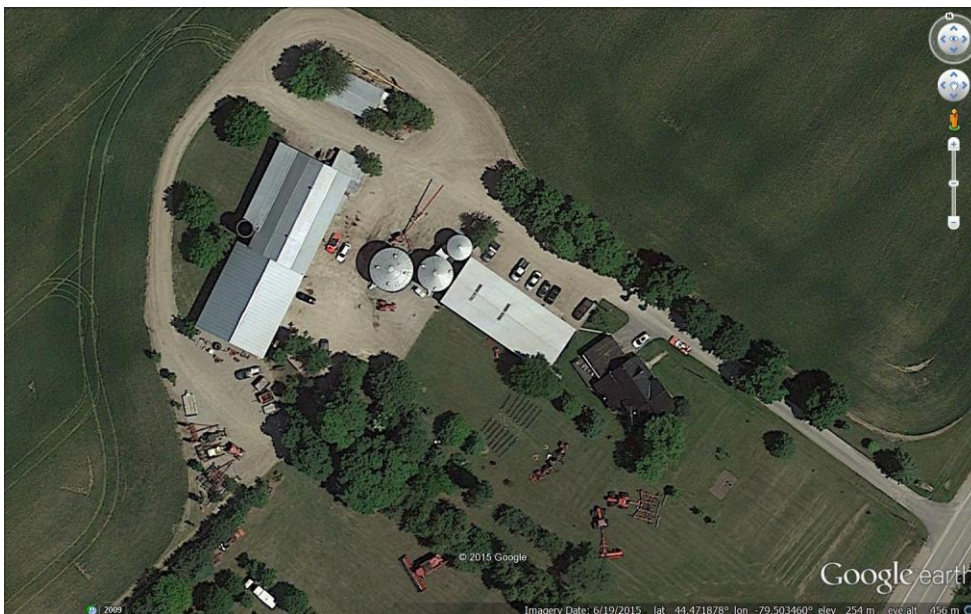
Agricultural Facility #8 – residential unit/garage, machine shed, bank barn with pole barn extension, shed, three grain bins, concrete silo (open top)
