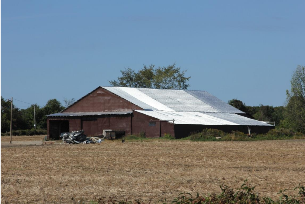
Agricultural Facility # 11 – residential unit, metal sided riding arena
