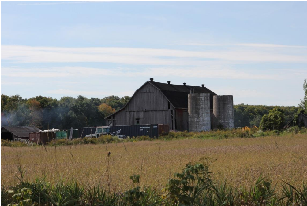
Agricultural Facility # 14 – Bank barn with extension (missing wall boards), two concrete silos (open top), three sheds (poor condition)
