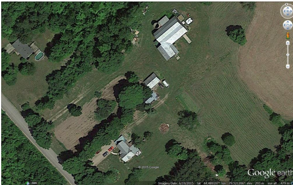
Agricultural Facility # 17 – bank barn with extensions, concrete silo (open top), sheds, residential unit
