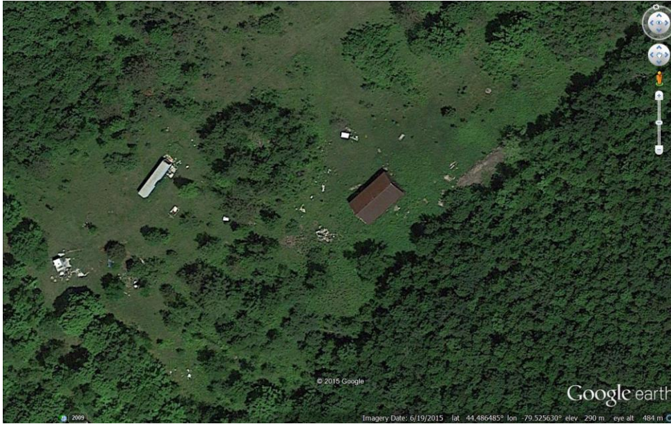
Agricultural Facility # 18 – pole barn
