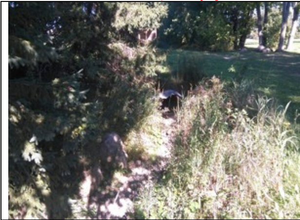
IMAGE 25 DISTURBED – SHOWS CULVERT & DITCH
