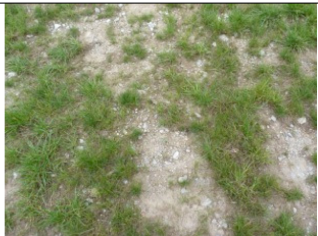
IMAGE 52 TEST PIT SURVEY CONDITIONS
