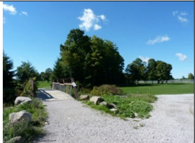
IMAGE 34 DISTURBED – SHOWS GRAVEL LANEWAYS & BRIDGE STRUCTURE
