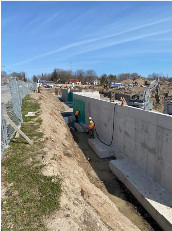
Continuation of exterior wall waterproofing.
