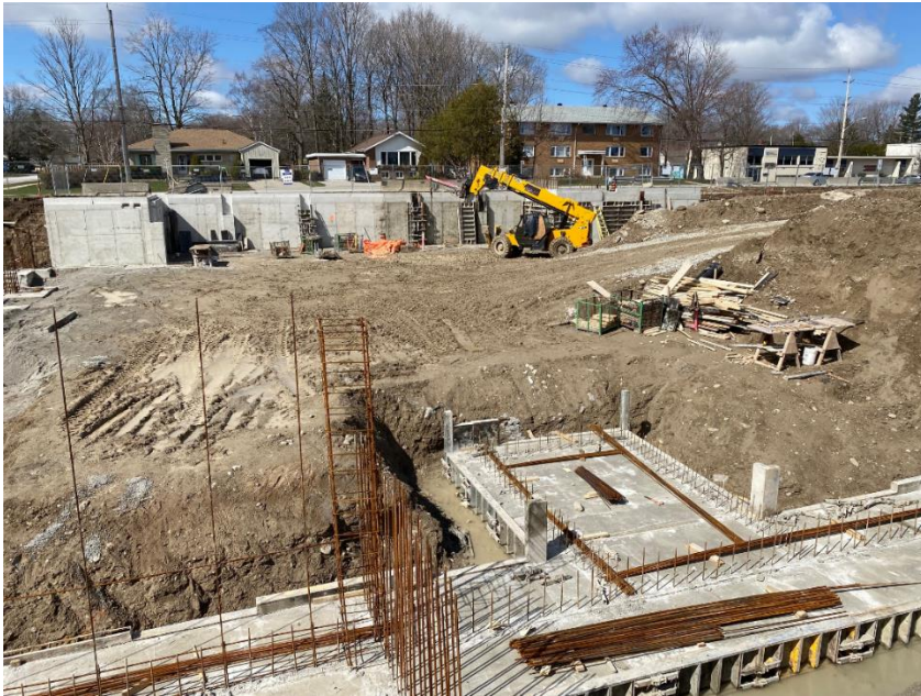
View looking towards West Street.
