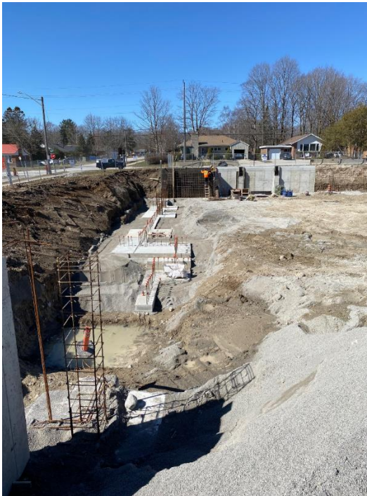
Foundation and walls being constructed in the hub basement.
