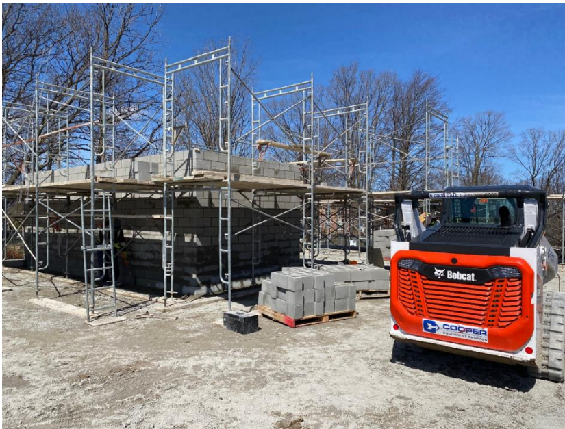
Stair D raising out of the ground.
