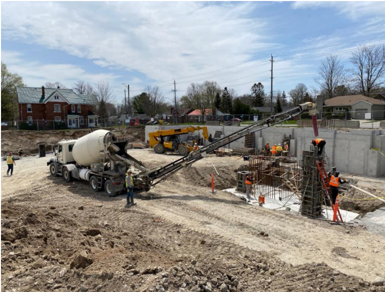
Pouring of columns and step footings for Stair B.
