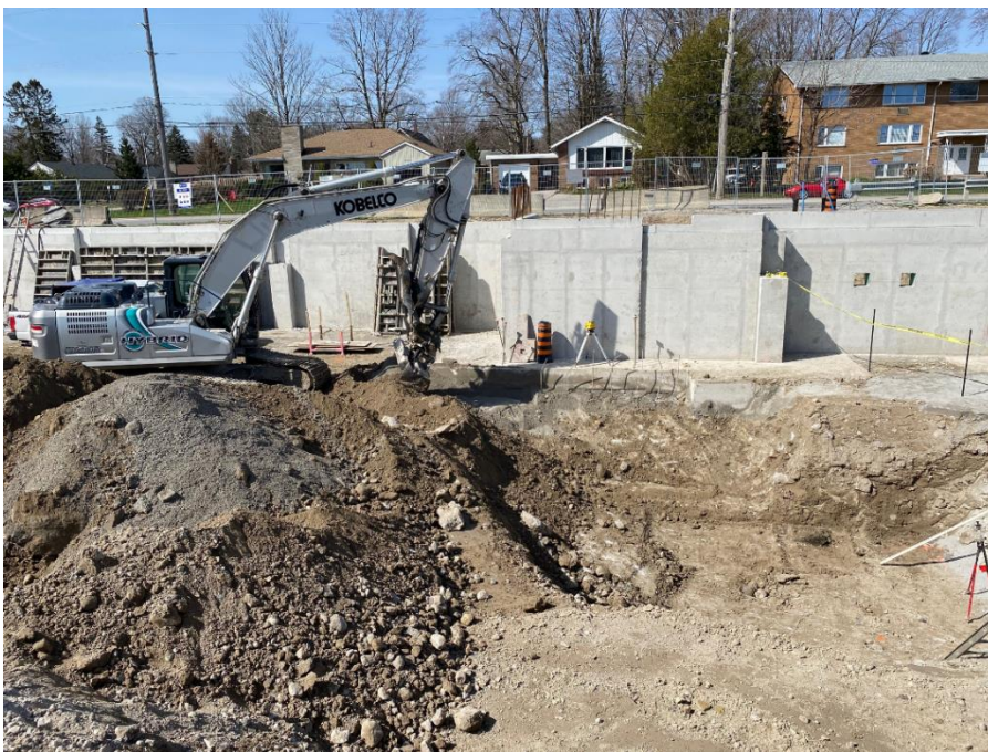
Continuation of the elevator pit excavation.
