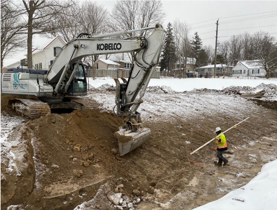
Start of construction on the storm water management pond
