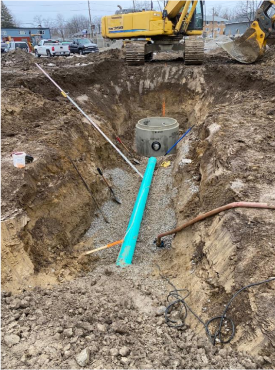
Storm and Sanitary Underway
