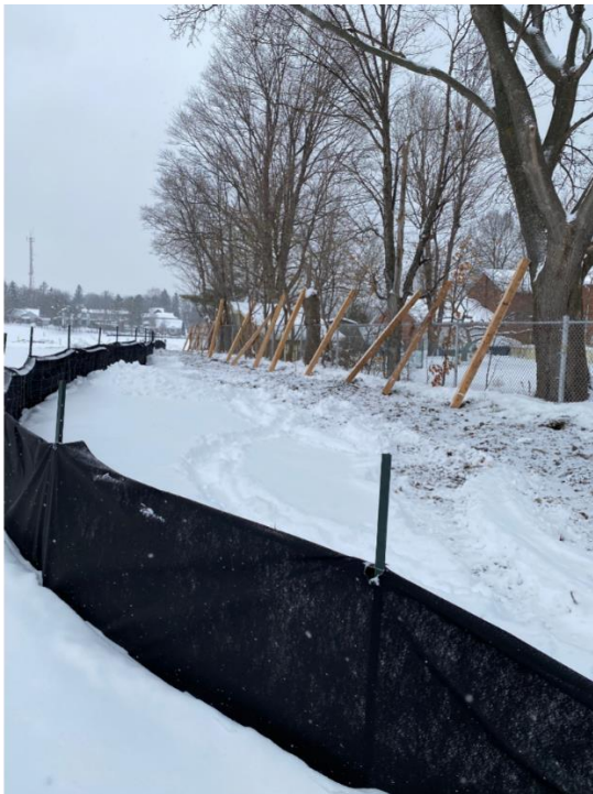
Wood Privacy Fencing and Silt & Erosion Fencing Underway
