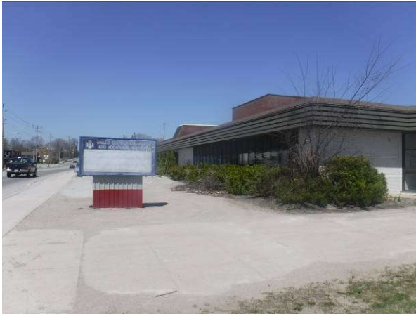
Plate 1: View from southwest corner of property looking along west side of school.
