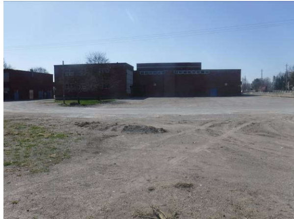
Plate 2: View across paved surface toward school.
