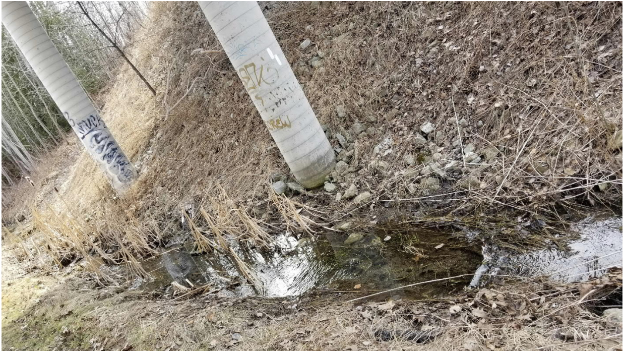
Photo 5: Creek underneath Old Fort Bridge
