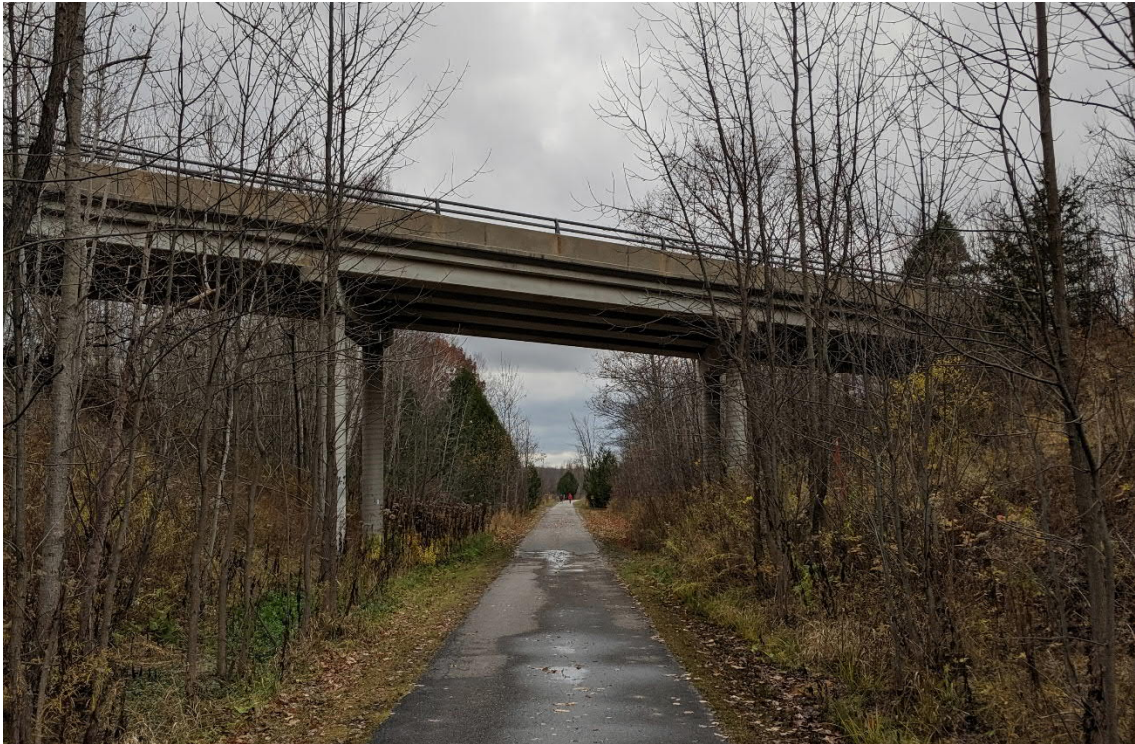
Photo 1: Old Fort Overhead Bridge (elevation looking west from trail)
