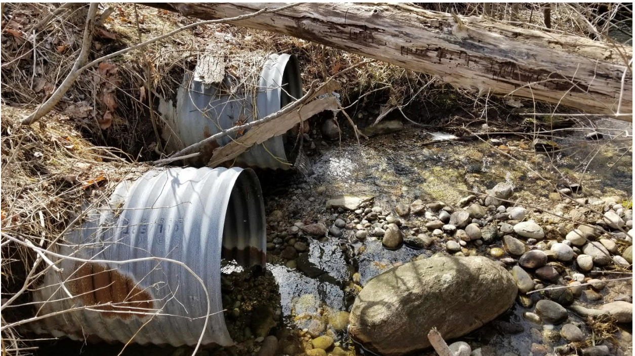
Photo 6: CSP culvert outlet on north west side of Old Fort Road
