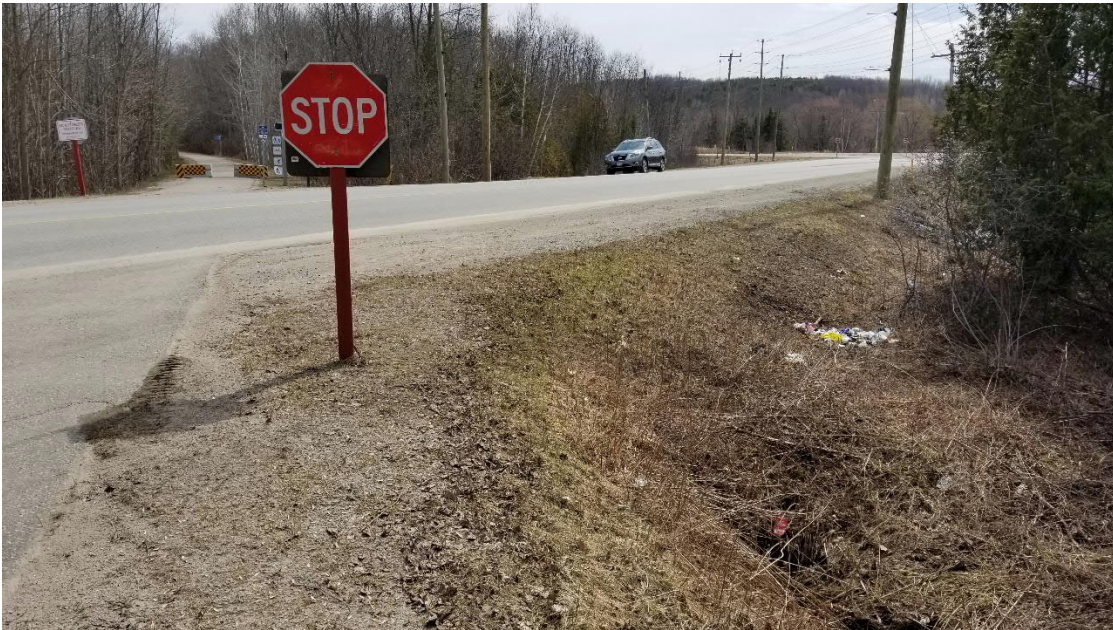
Photo 8: General view of at-grade crossing at Triple Bay Road and Trans Canada Trail
