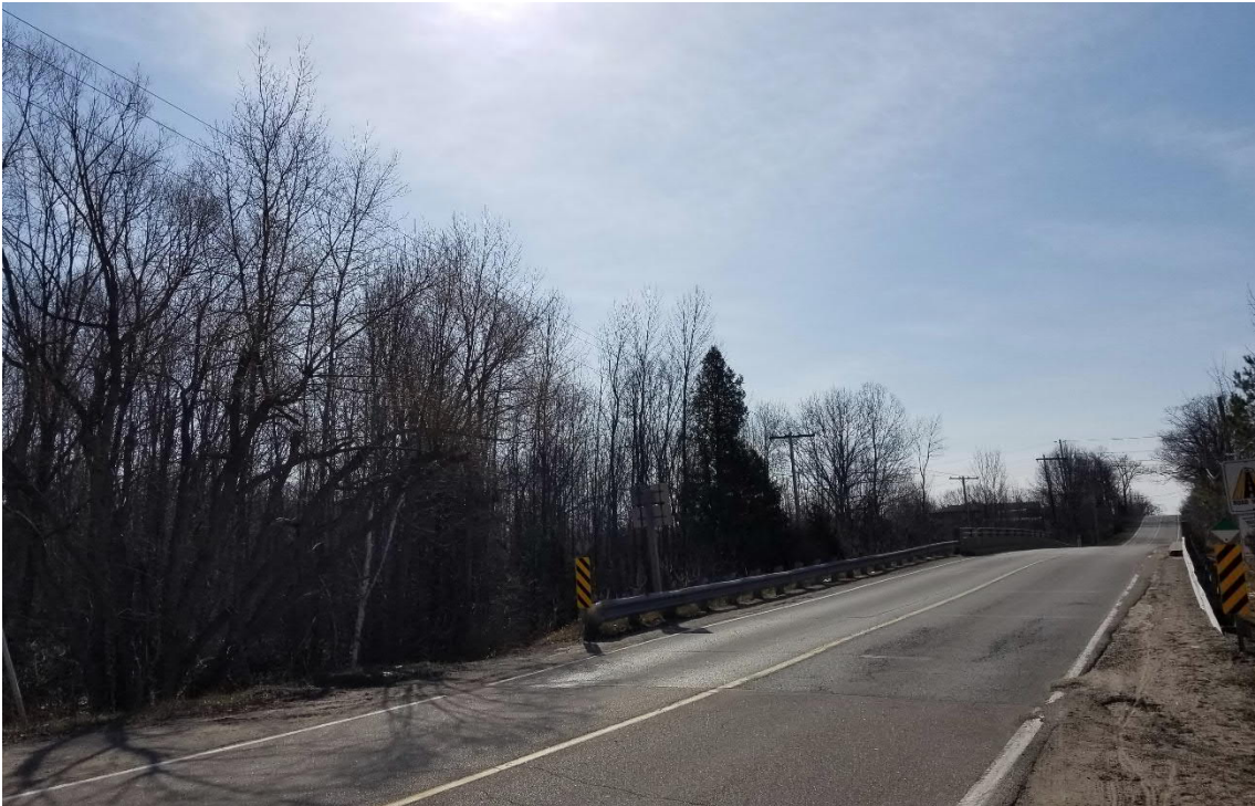
Photo 2: Old Fort Road, bridge north approach looking south
