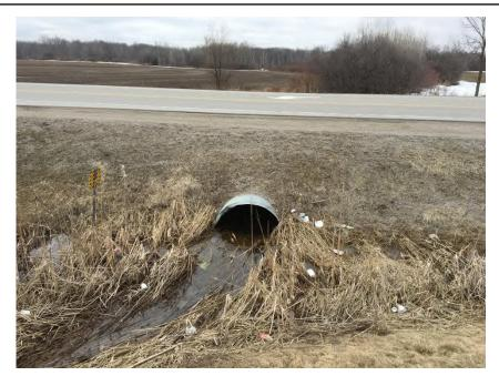
**Photograph 11:** North CSP culvert crossing of County Road 53 (conveying the Lawson Drain) within the Study Area (facing west at culvert outlet; March 25, 2020).
